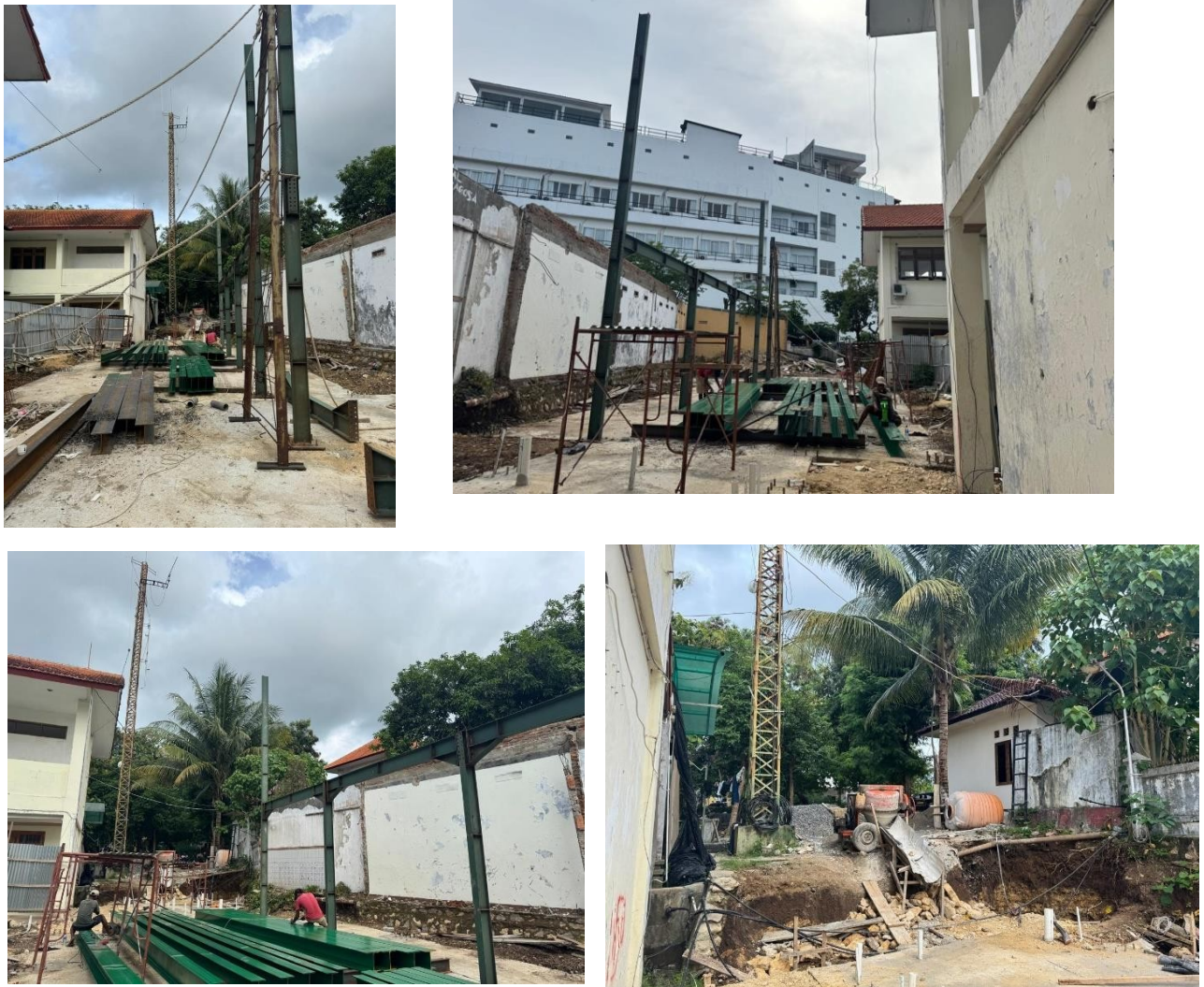
Figure 9. Renovation and Expansion of the Office Building
